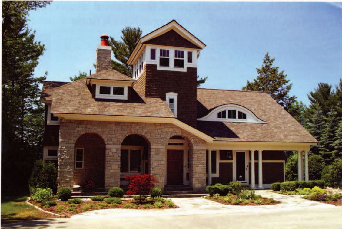
Inspired, Ken VanHouten strives for the absolute best in design, combining true innovation and uncompromising quality that captures a homeowner's discriminating tastes and lifestyle in a custom home that delivers a statement. Elements of distinction are a Fish-eye window and a European style Tower loft surrounded by energy efficient windows offering an intimate escape.
